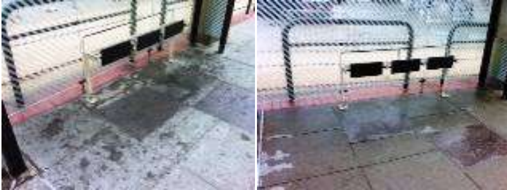
September 12, 2011: Jan Warner Plaza, scrub within the bus shelter completed
