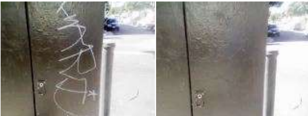
September 26, 2011: 153 Sanchez St. Graffiti Removed
