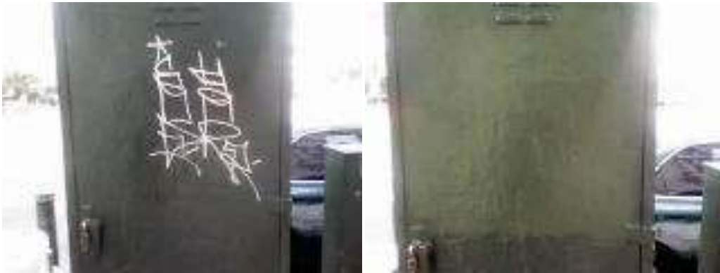
October 16, 2011: 2099 Market St. Graffiti Removed
