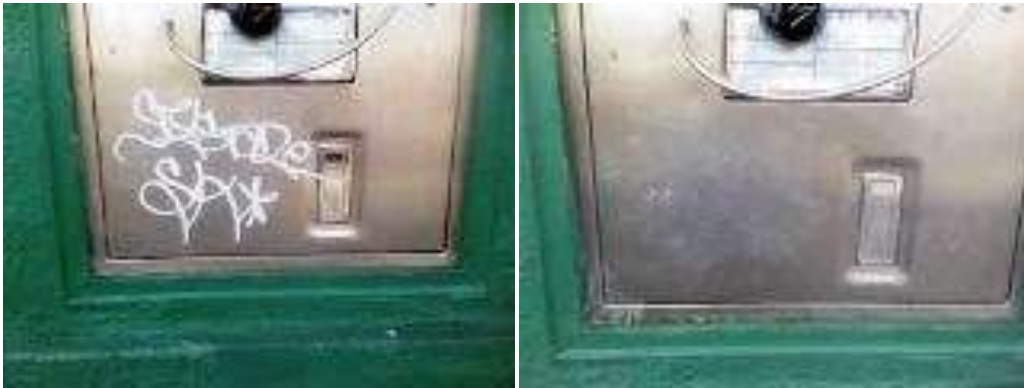
October 25, 2011: 1946 Market St. Graffiti Removed
