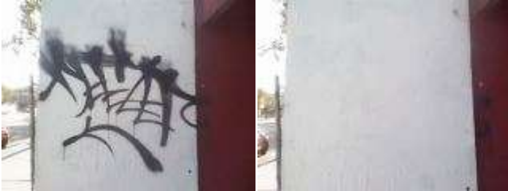
October 28, 2011: 1800 Market St. Graffiti Removed
