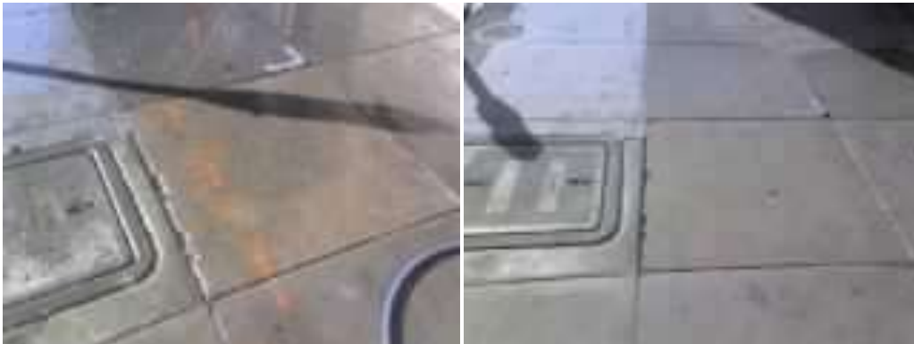
October 15, 2011: 446 Castro St. Steam Clean Completed
