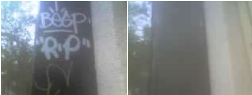
October 9, 2011: 2100 Market St. Graffiti Removed
