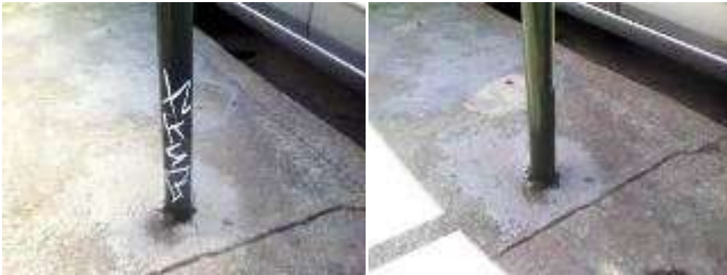
October 11, 2011: 1939 Duboce St. Graffiti Removed
