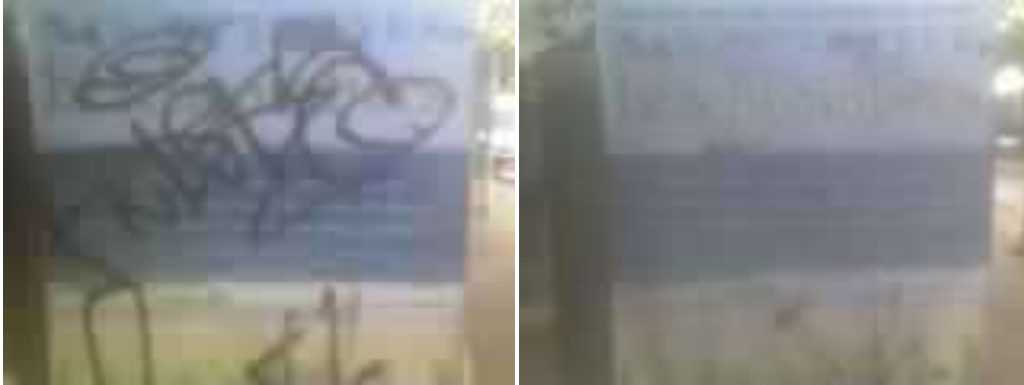
October 11, 2011: 2370 Market St. Graffiti Removed
