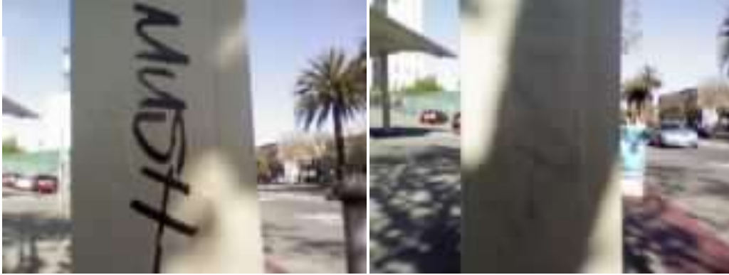
October 27, 2011: 1967 Market St. Graffiti Removed
