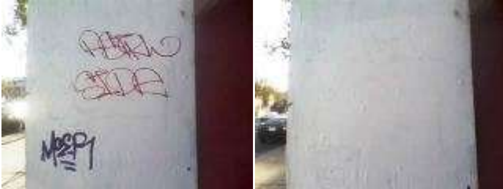
October 23, 2011: 1800 Market St. Graffiti Removed
