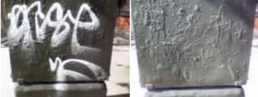
October 19, 2011: 1800 Market St. Graffiti Removed
