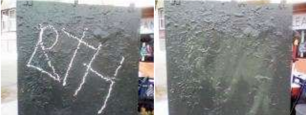
October 2, 2011: 1890 Market St. Graffiti Removed
