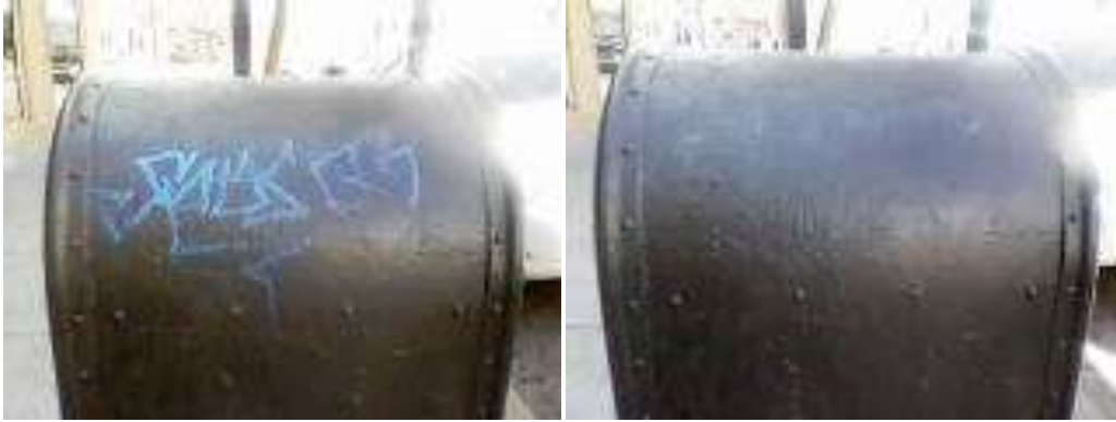
October 9, 2011: 1939 Market St. Graffiti Removed
