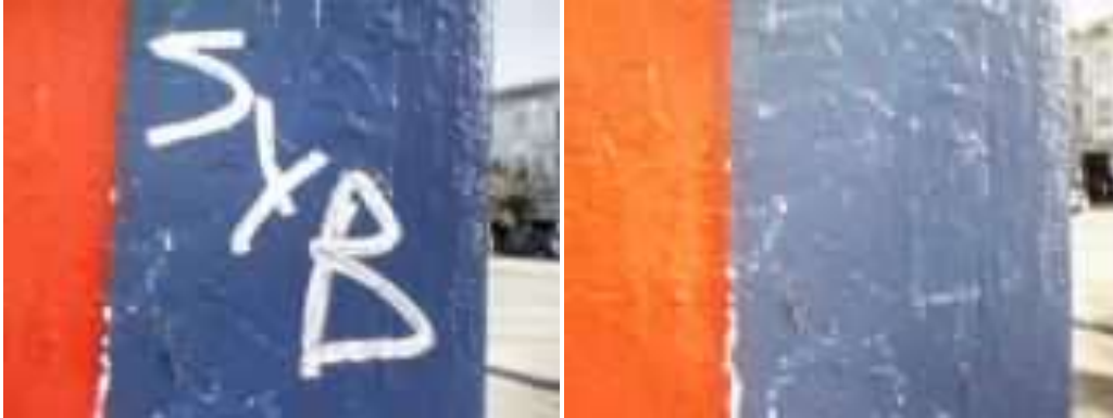
October 21, 2011: 2100 Market St. Graffiti Removed
