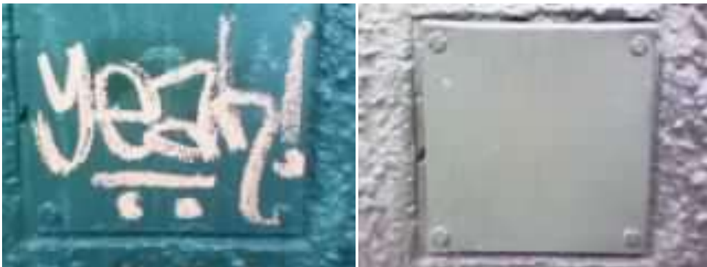
October 19, 2011: 1975 Market St. Graffiti Removed
