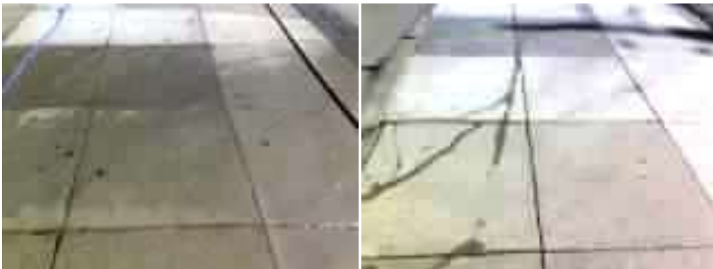
October 8, 2011: 17 th St Market to Hartford St. Steam clean completed
