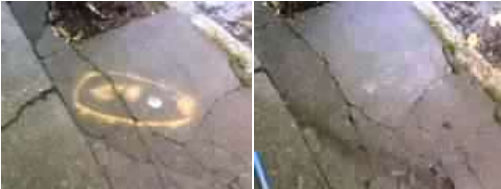
May 16, 2011: Pond near 17 th St. Steam clean completed
