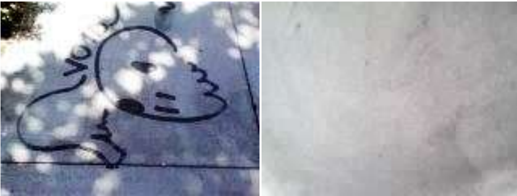
May 20, 2011: 153 Sanchez St. Graffiti Removed
