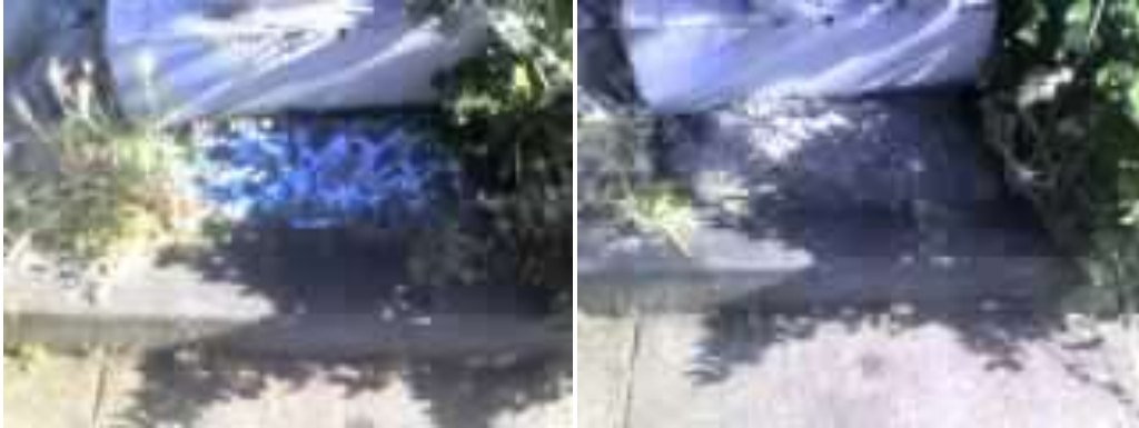
May 2, 2011: 2174 Market St. Steam clean completed
