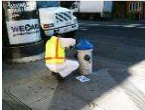
May 4, 2011: DPW painting hydrants on Castro St.
