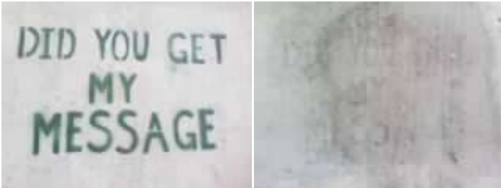
June 16, 2011: 698 14 th St. Graffiti Removed
