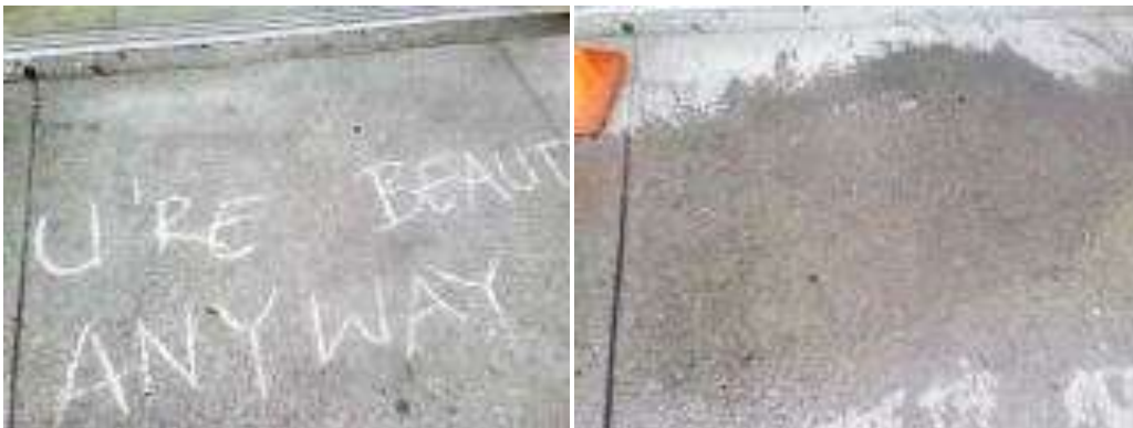
June 27, 2011: 2301 Market St. Graffiti Removed
