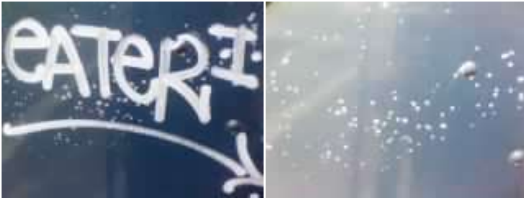
June 8, 2011: 2099 Market St. Graffiti Removed
