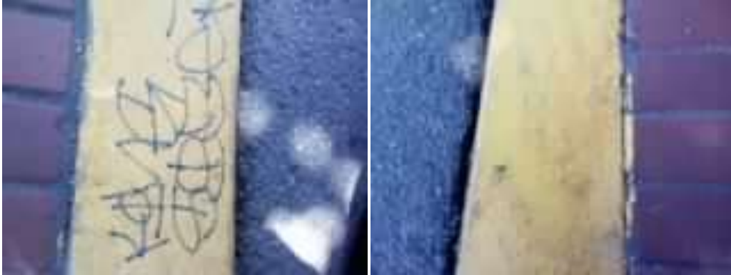
June 9, 2011: 1815 Market St. Graffiti Removed
