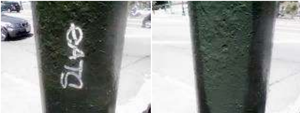
June 12, 2011: 1965 Market St. Graffiti Removed
