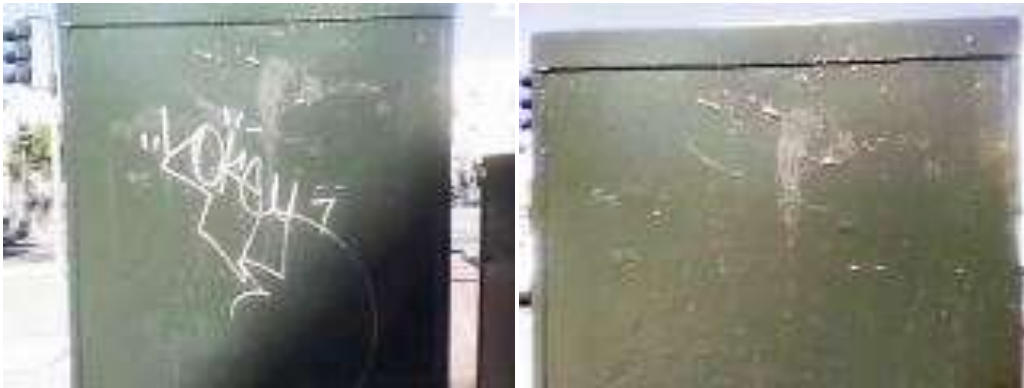
June 14, 2011: 1800 Market St. Graffiti Removed
