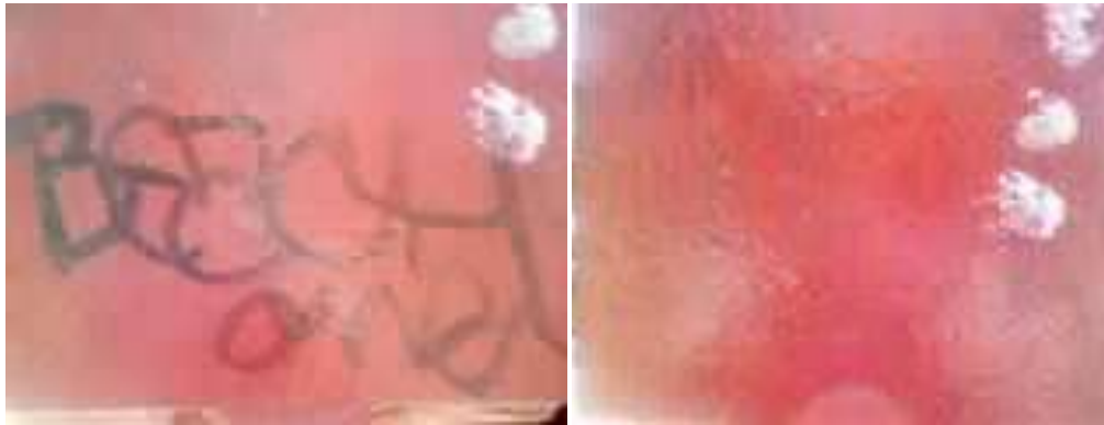
June 27, 2011: 2201 Market St. Graffiti Removed
