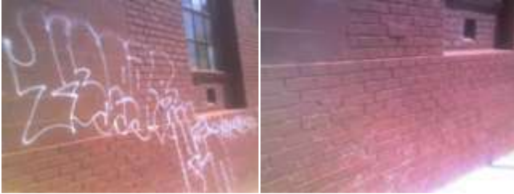
June 7, 2011: Rear of 2355 Market St. Business provided paint, removal completed
