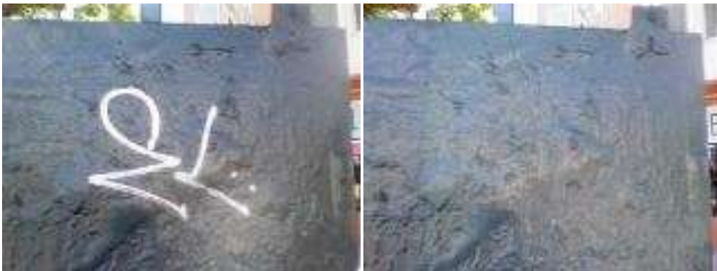
June 14, 2011: 1890 Market St. Graffiti Removed
