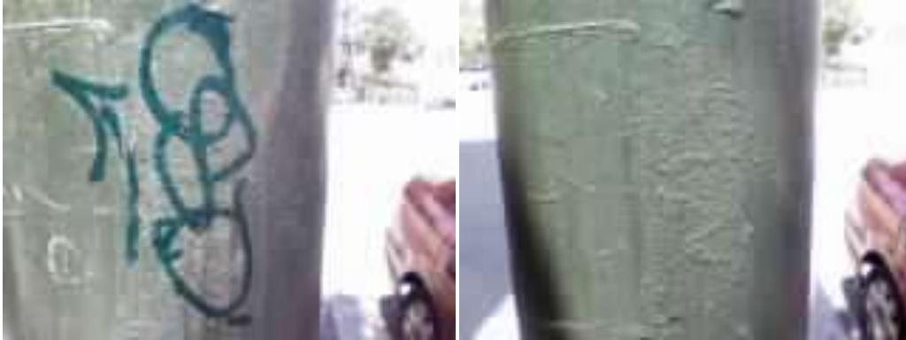
June 2, 2011: 1900 Market St. Graffiti Removed
