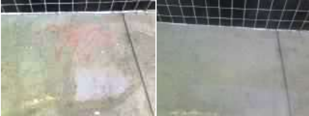
August 11, 2011: 1906 Market St. Steam clean completed
