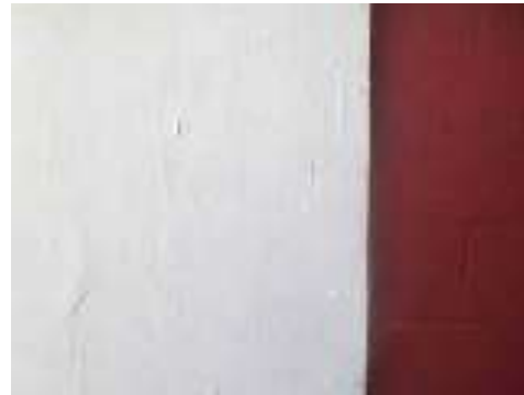
After restriction removed
