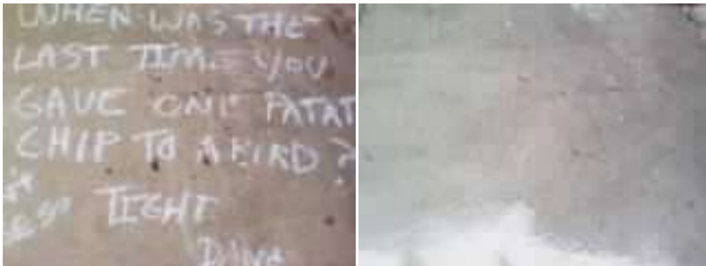
August 27, 2011: 431 Castro St. Graffiti Removed
