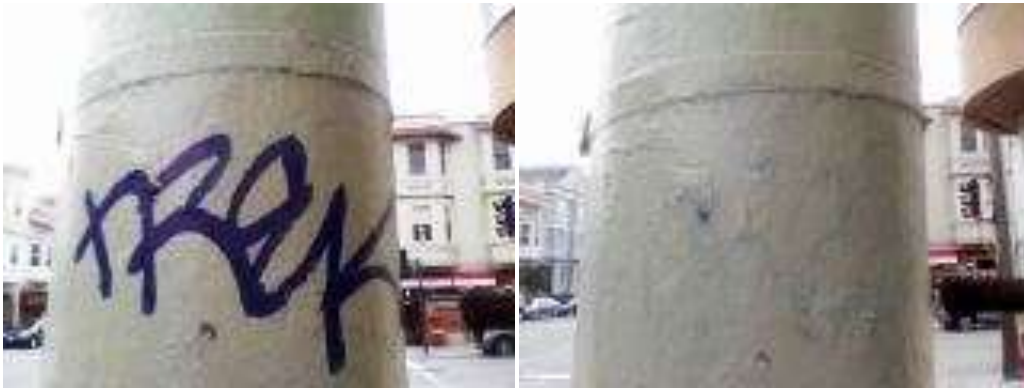
April 17, 2011: 296 Church St. Graffiti Removed
