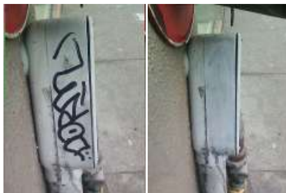
April 22, 2011: 4071 18 th St. Graffiti Removed
