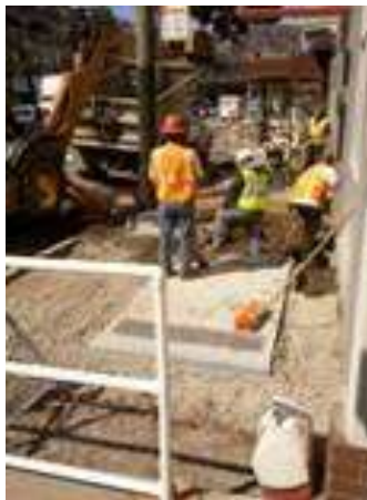
541 Castro construction work closes sidewalk and curb area
