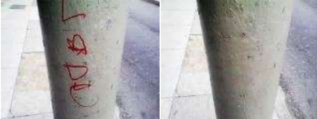
April 18, 2011: 225 Church St. Graffiti Removed
