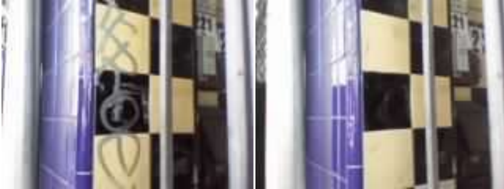
April 6, 2011: 223 Church St. Graffiti Removed
