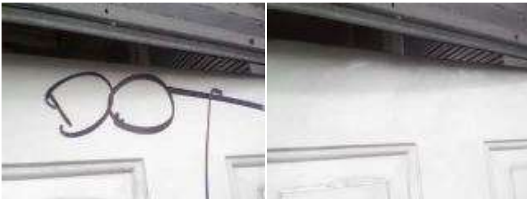
April 19, 2011: 242 Church St. Graffiti Removed
