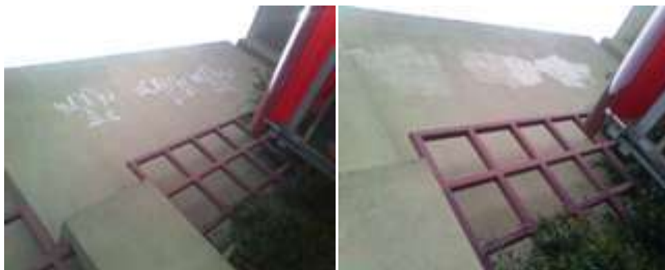
April 22, 2011: 100 Church St. Graffiti Removed
