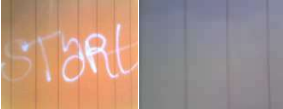
April 19, 2011: 2200 15 th St. Graffiti Removed
